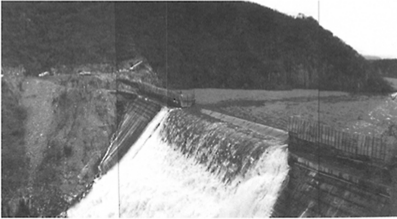
Figure 4. Skimming flow down Trigomil stepped spillway (Mexico): Q_w=1,017 \text{ m}^3/\text{s} , chute width: 75 m (Courtesy of Drs Sanchez-Bribiesca and Gonzales-Villareal).
